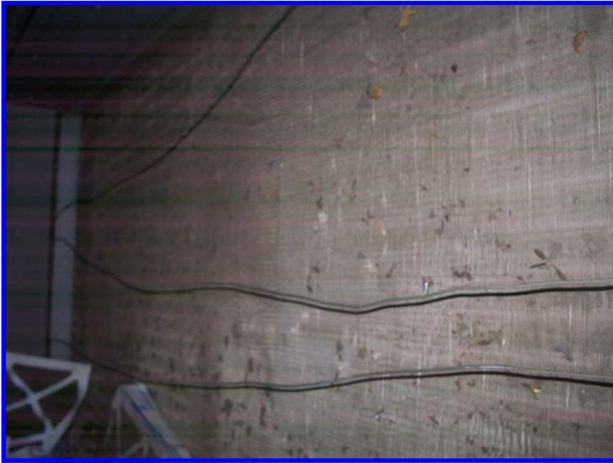
WEIGHT ROOM-UNIT COIL
