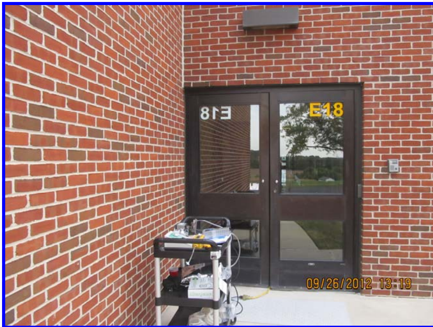
SAMPLE LOCATION ROOM # 135
